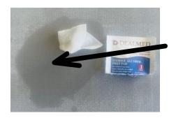
1st begin by preparing the area where you plan to adhere your Sink Clip, by taking an alcoholic swab and gently cleaning the area of any dust or residue left after fabrication
